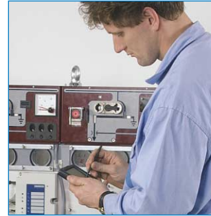
Easily adjustable electronic protection relay.
