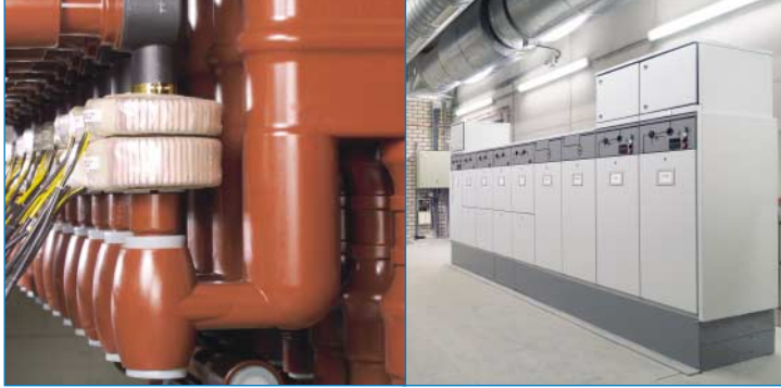
Current transformers type CTS as used in Innovac SVS.
